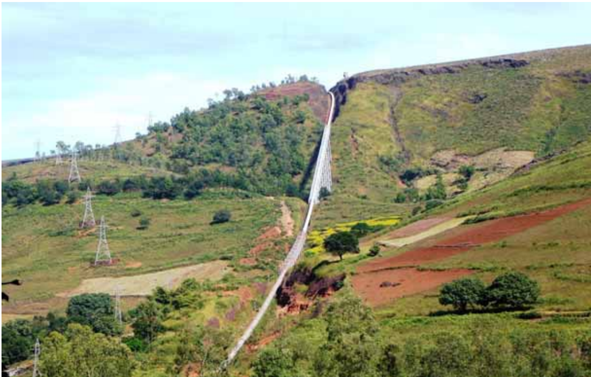
Conveyor Belt of Nalco plant
