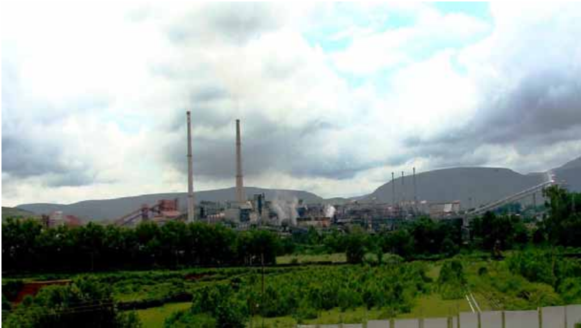
Nalco plant at Damanjori
